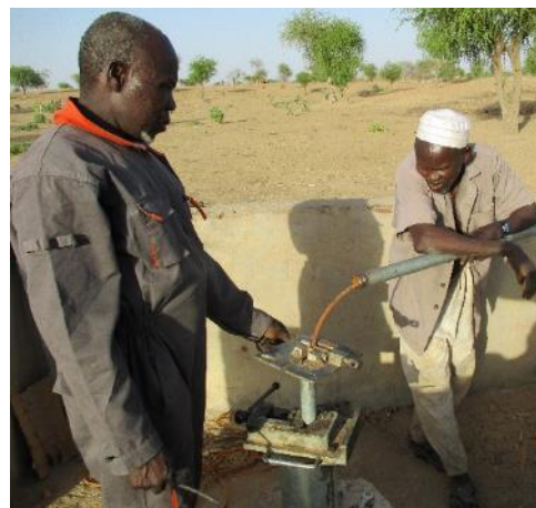
Figure 5 –Replacing the pump at Hille Tahir Village
