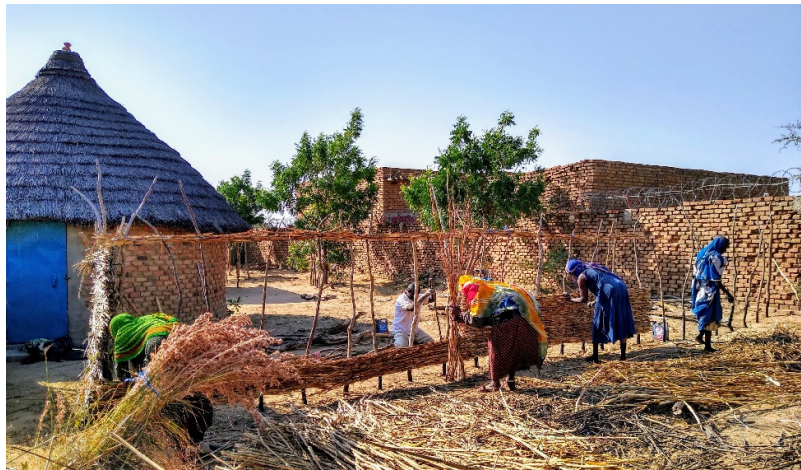
Figure 3: Building a new tar tar wall next to one of the SAS guest huts.
